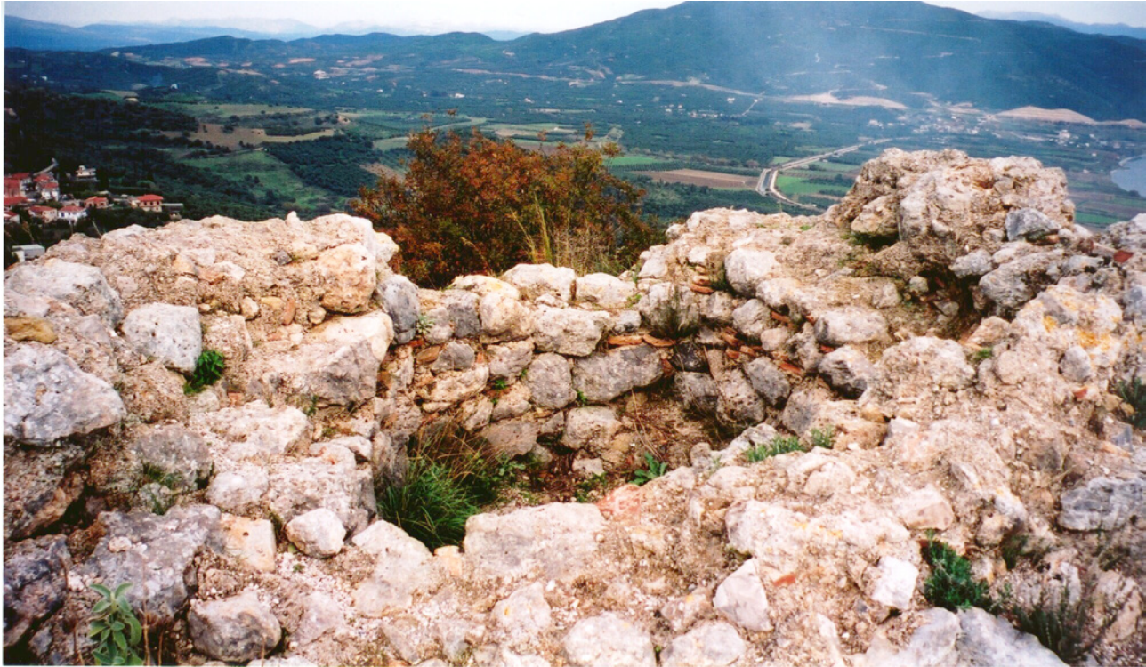
Fig. 100. Ag. Ilias, tower. View of the interior from the S.
